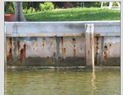
Typical concrete panels.
